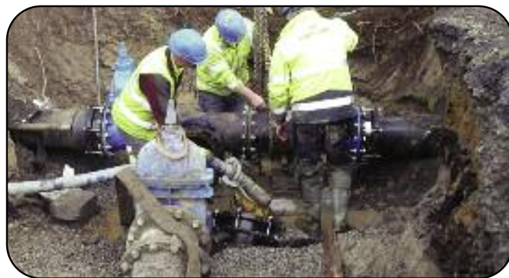
Portlaoise RAL project - Pipe laying in Shaen
