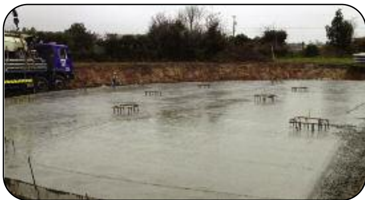
Construction of Knocks Reservoir
