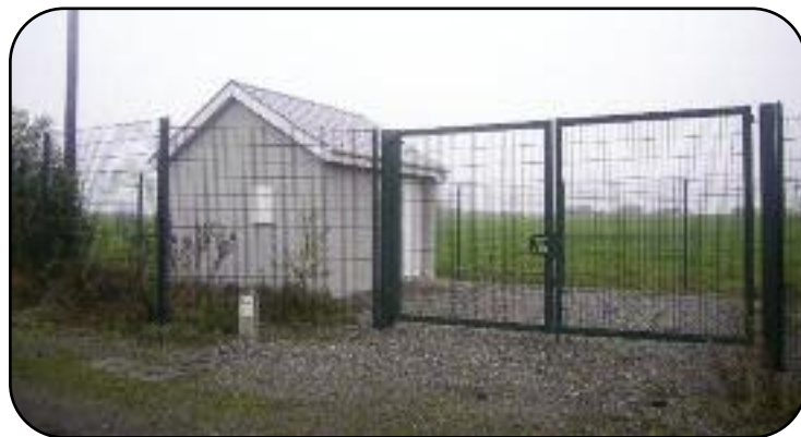
Reary Pumphouse upgraded in 2013
